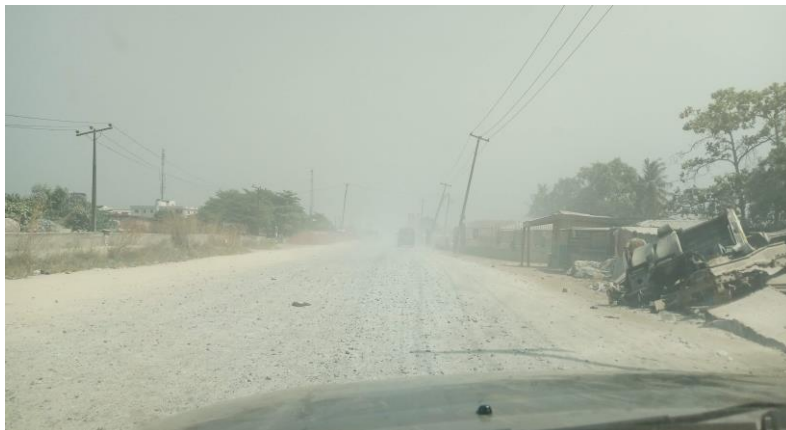
Plate 8: Poor dust control around a construction site in Nigeria
