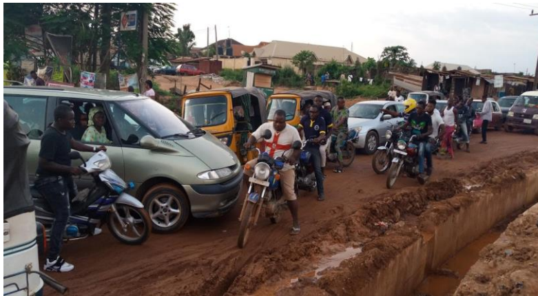
Plate 7: Poor Traffic Management around a construction site in Nigeria
