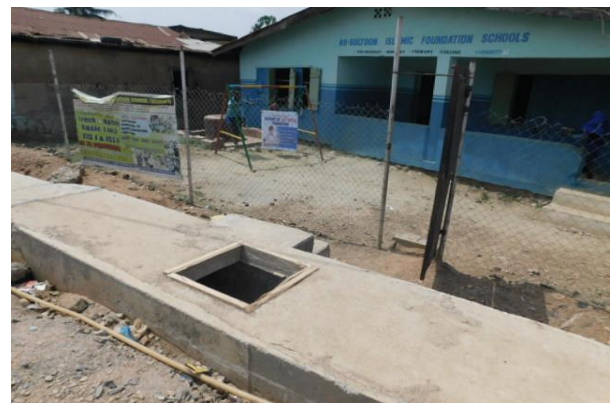
Plates 3 and 4: Protruding reinforcements and Open manholes along drains for road construction projects
