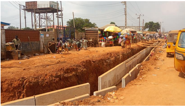
Plates 1 and 2: Poor temporary access provision around road construction sites in Nigeria
