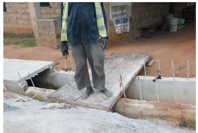
Plates 5 and 6: Workers on a Construction site without appropriate PPEs
